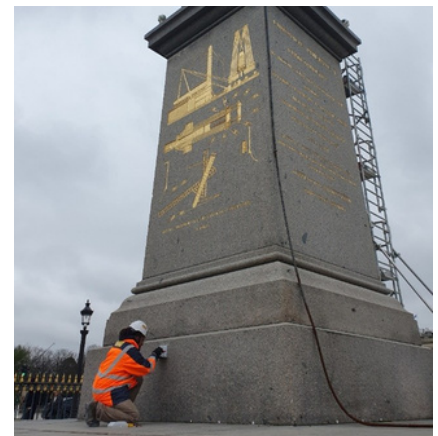
Figure 4: Luxor Obelisk with the installation of the SHM SYSCOM ROCK Acceleration device
