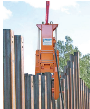
Figure 1. Pajot 2800 hammer used for piling
