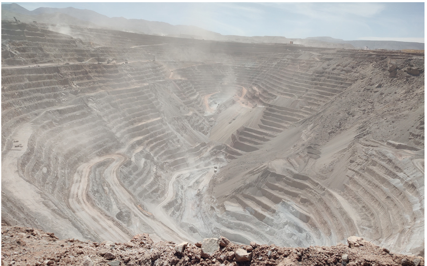
Figure 1. View of the DMH open pit mine with the big collapse in the right part.
