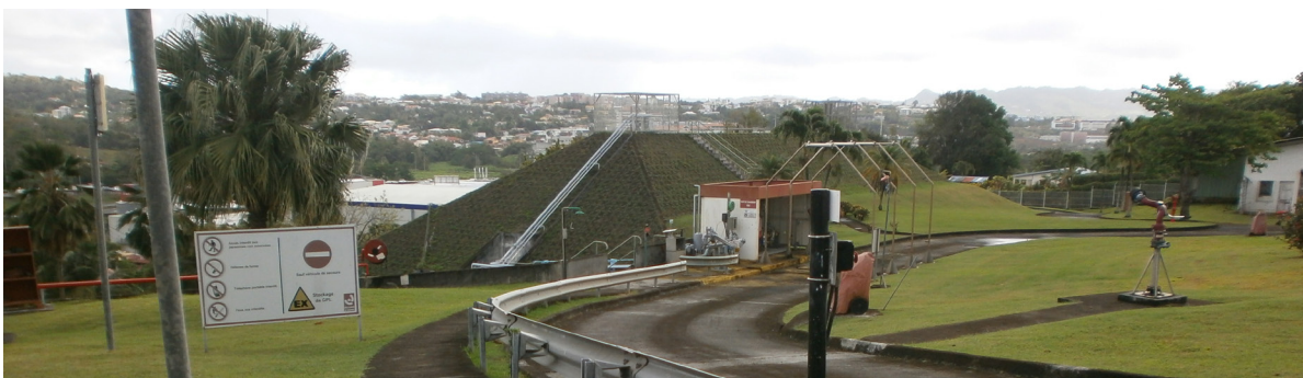
Figure 4. Site view with LNG Tank under slope
