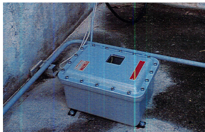
Figure 1. MRSK in Ex d enclosure
