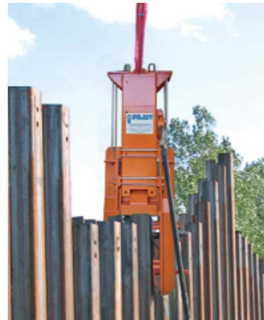
Figure 1. Pajot 2800 hammer used for piling
