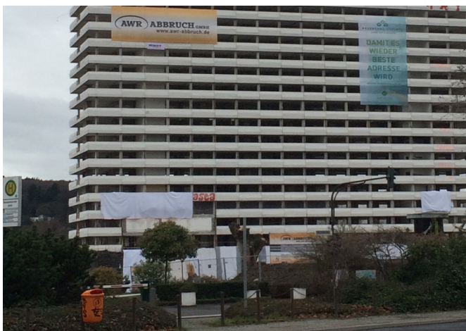
Figure 1. The Bonn Center few minutes before the demolition.
