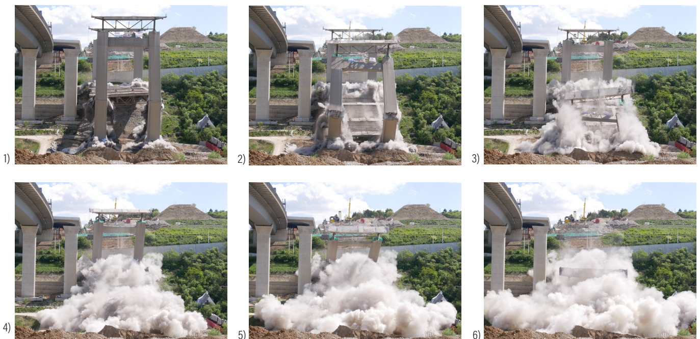
Figure 3. Successive frames of the bridge demolition.
