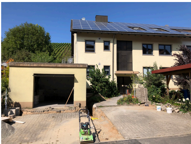
Figure 2: Exterior view of the residential building
