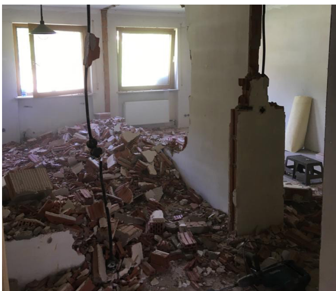
Figure 4. Demolition works on the first floor.
