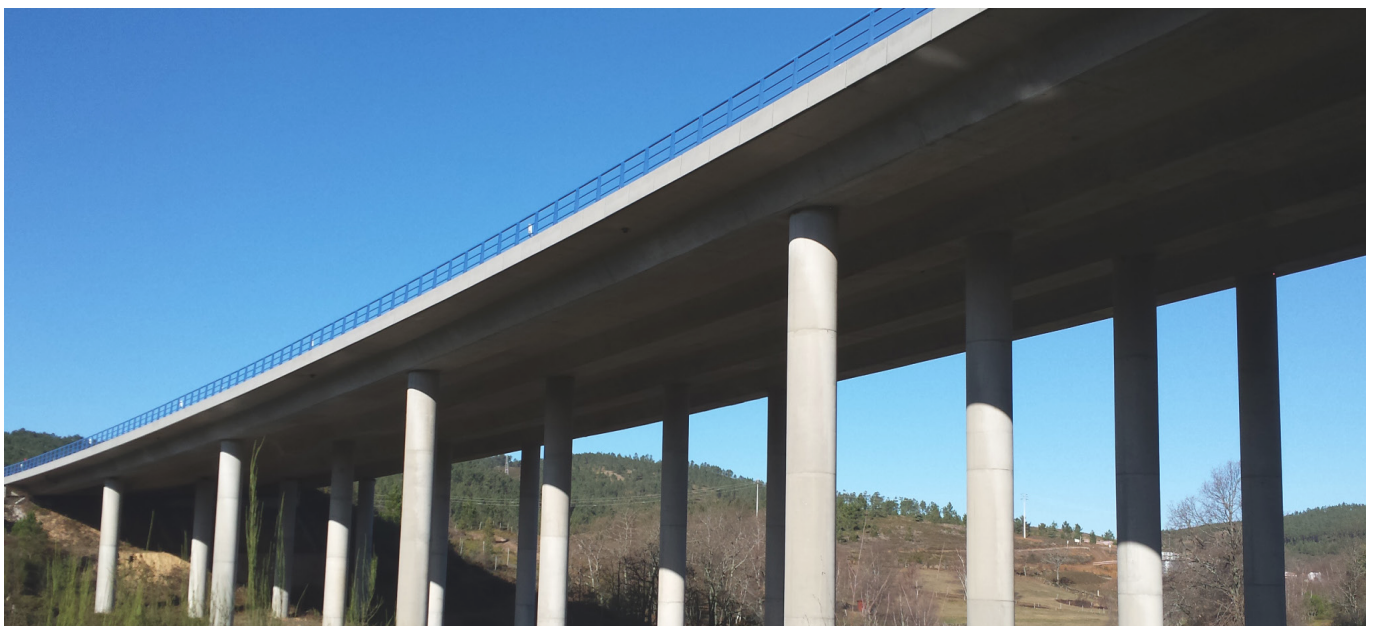
Figure 1. The A7 viaduto bridge, in the north part of Portugal.
