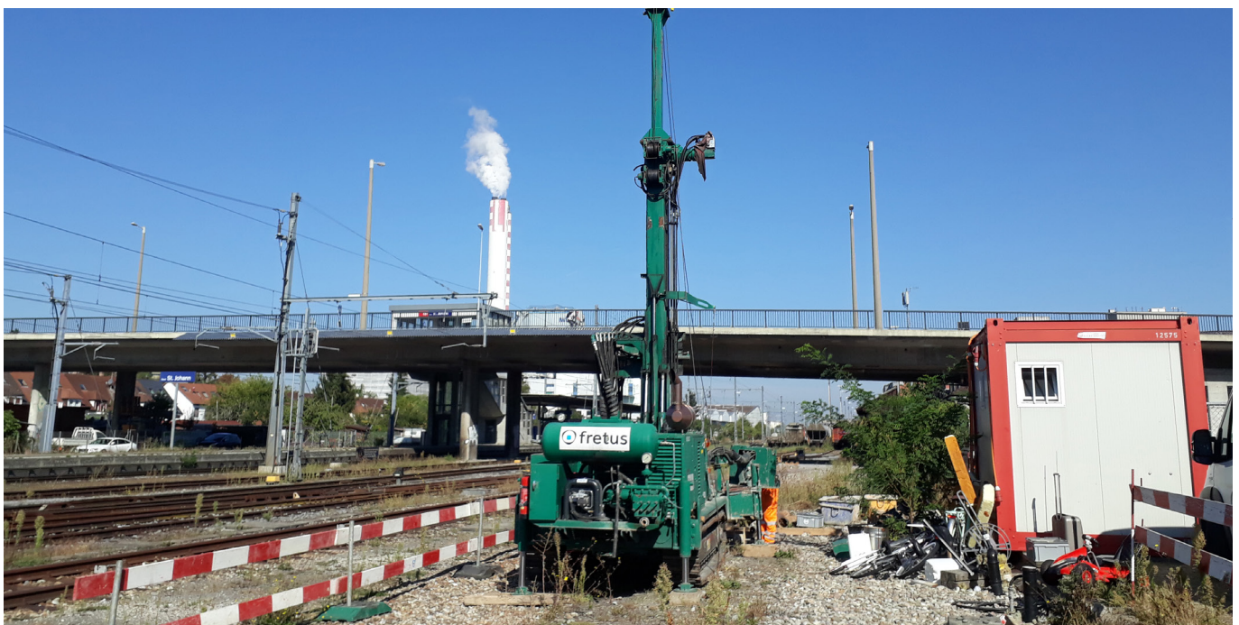
Figure 2. The construction site with a driller machine.
