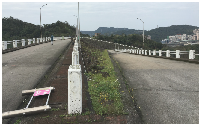
Figure 5. View of the dam from the main entrance of the control center.
