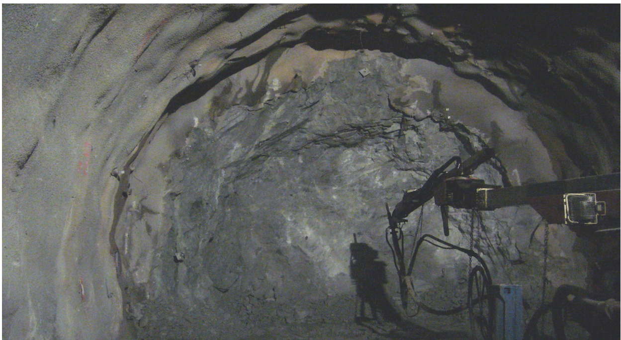
Figure 1. Preparation of boreholes for blast excavation.
