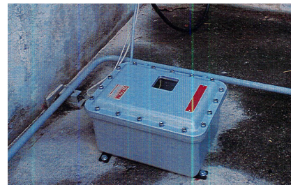
Figure 1. MRSK in Ex d enclosure
