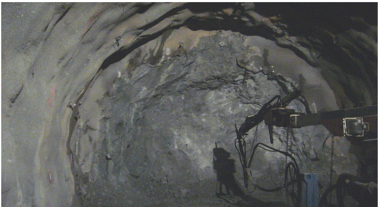
Figure 1. Preparation of boreholes for blast excavation.
